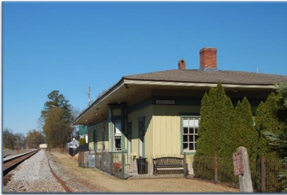
Adairville W&A Depot, Bartow County
