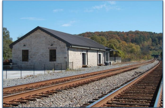
Tunnel Hill W&A Depot, Whitfield County. New tunnel for modern railroad can be see at right in the distance.
