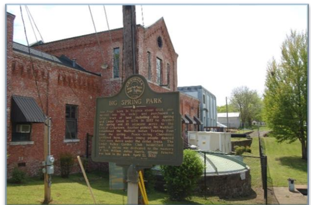
Big Spring Waterworks building, Cedartown
