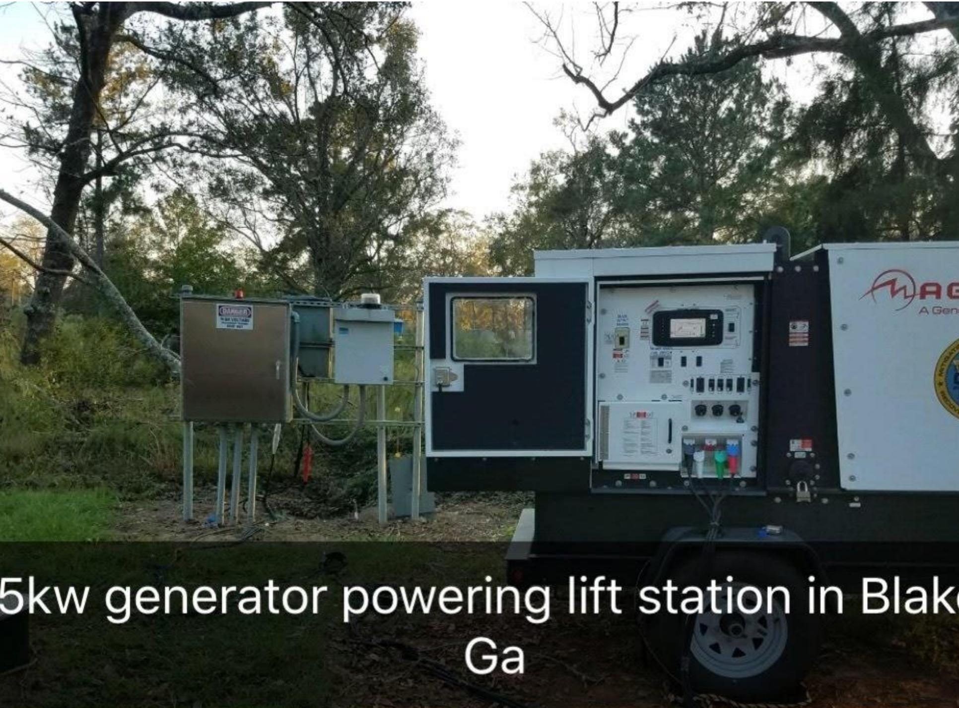
5kw generator powering lift station in Blak
