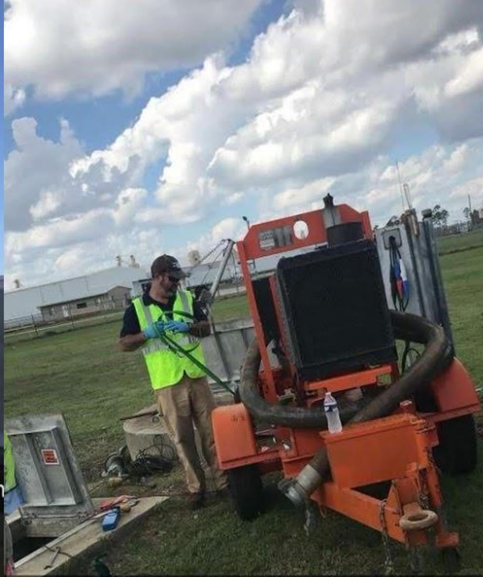
Bypass pump from Zebulon Ga being put in at Donalsonville lift station
